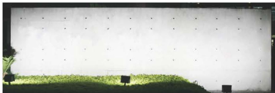
Distance between luminaires : 1.5m-2.5m
