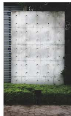
Distance between luminaires : 1m-1.5m
